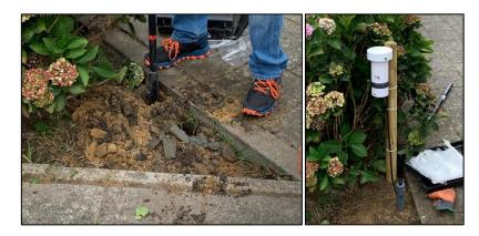
Figures 4 and 5: installation of the soil moisture, humidity and temperature sensors used in the SCOREwater project. On the picture we see digging of the hole where the soil moisture sensor is placed (left), and a measuring unit used by Measure Your City (right).
